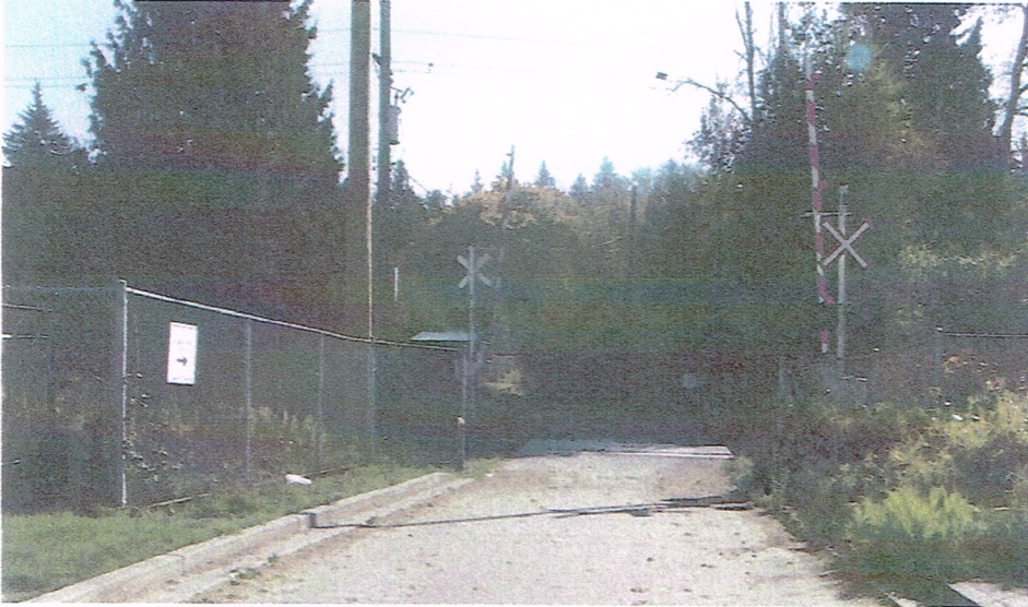
Figure 13.12 Existing Railway Crossing at Trinity Western University
