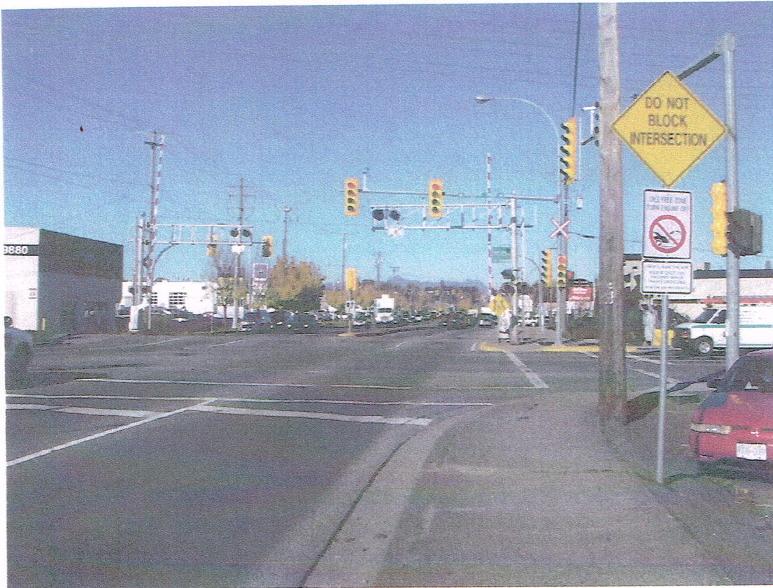
Figure 13.3 Existing Railway Crossing at 200th Street
