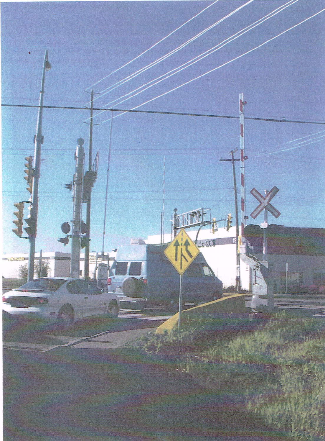
Figure 13.4 Existing Railway Crossing at 200th Street
