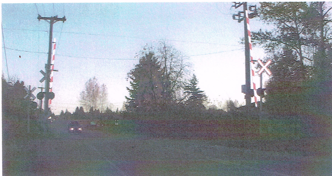
Figure 13.13 Existing Railway Crossing on 232 nd Street
