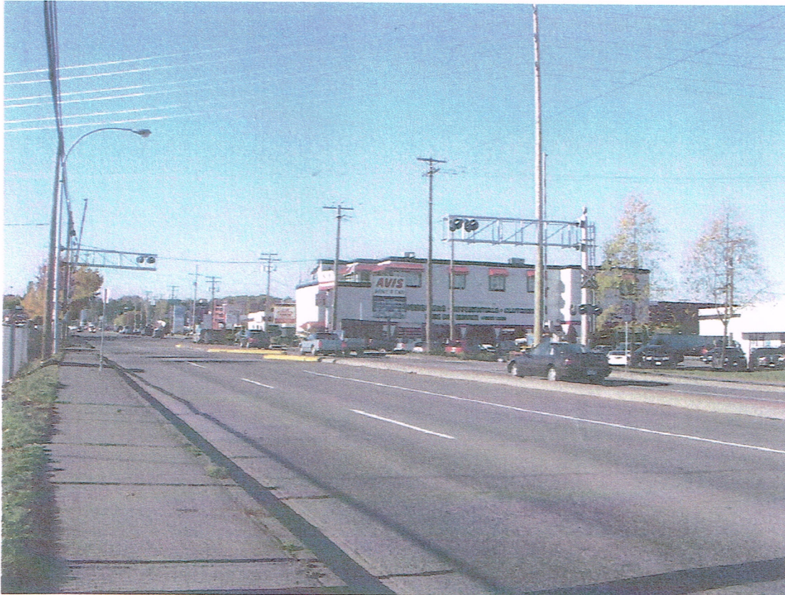
Figure 13.5 Existing Railway Crossing on Fraser Highway
