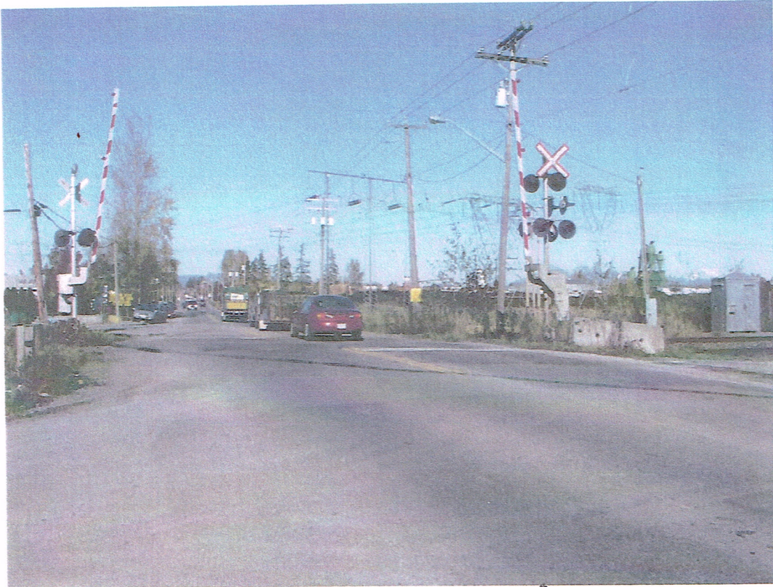
Figure 13.2 Existing Railway Crossing at 56 th Avenue
