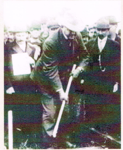
Premier Robert McBride driving the last spike at the Chilliwack terminus.
